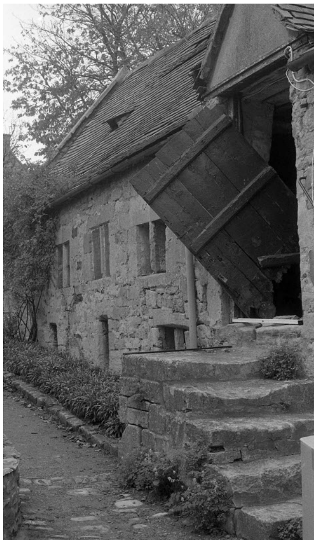
Fig. 1. The malthouse before work began, from the south east
