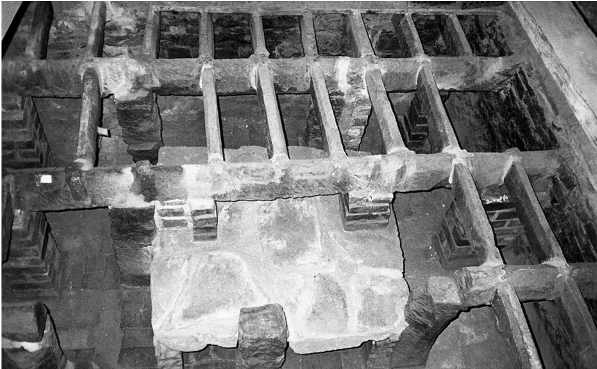
Fig. 9. Underside of stone grid showing underside of kiln tiles and some of the grid support pillars
