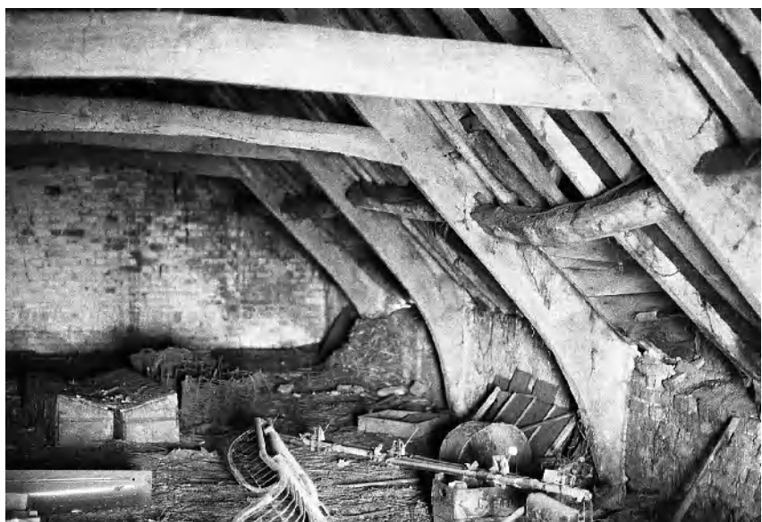
Figure 4 Interior - top floor showing roof structure
