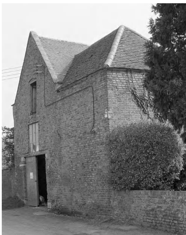
Figure 1 Kiln and malthouse from the south west
