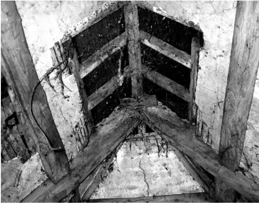
Figure 8 Interior kiln roof showing location of cowl
