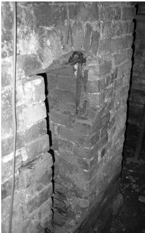
Figures 6 and 7 Kiln furnace mouth
