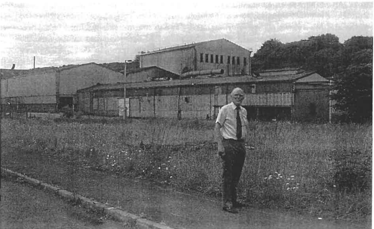
Lister-Peter Site Dursley. Peter Platt-Higgins (Ove Arup) in front of the former foundry
