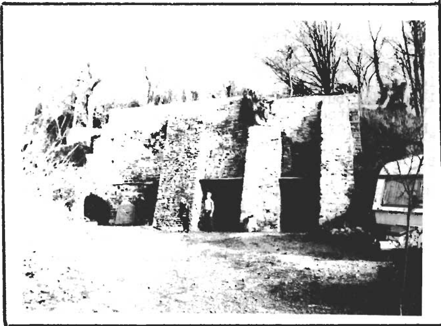
Rockland Kilns Recently restored and now used as garages. Corrugated iron over the entrances to two of the chambers obscures the view of the arches. (Photo - D. Bick)
