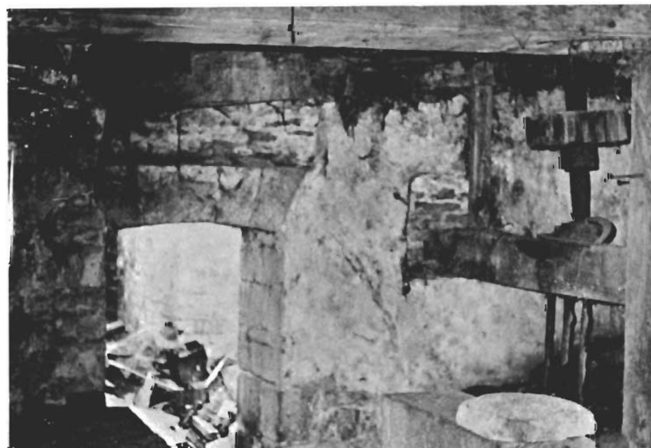
FLAXLEY MILL (20) THE HOLE FOR THE WATER WHEEL AXLE AND THE LEFT HAND STONE NUT
