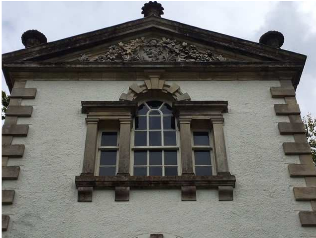
Detail of the tower's pediment, surmounted with what are thought to be the arms of the Shurmur family
