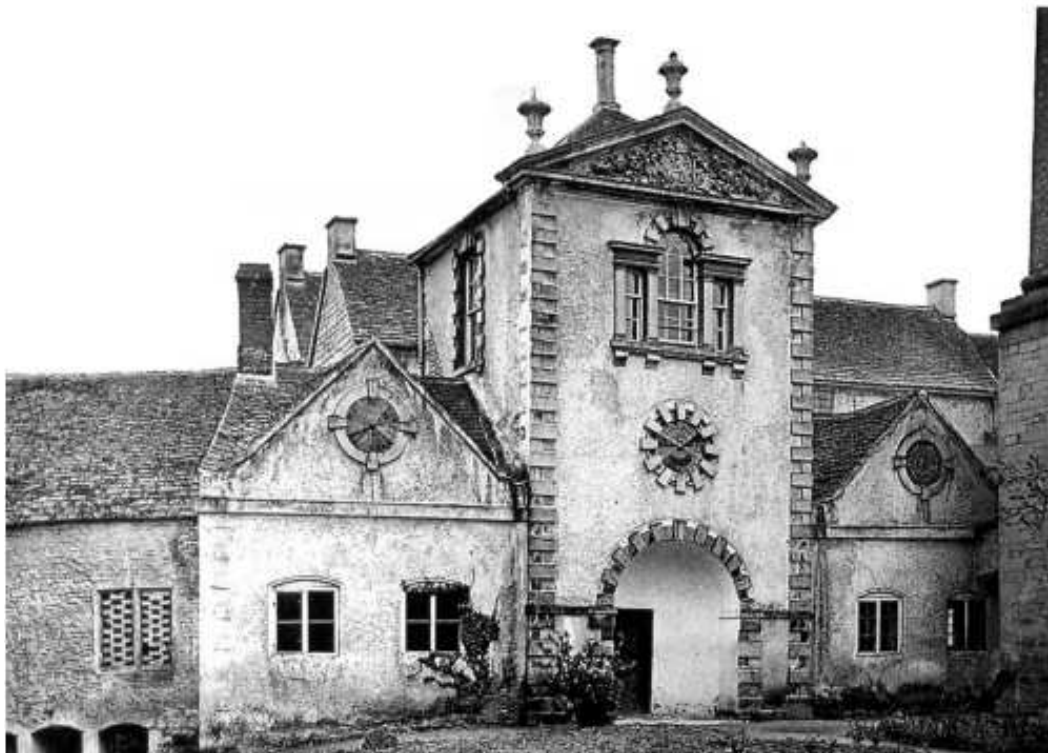
The Pin Mill in the 1930s. Note the central Venetian window and the dressed stone quoins. Also, that the original openings in the wings have been blocked up and replaced with windows
