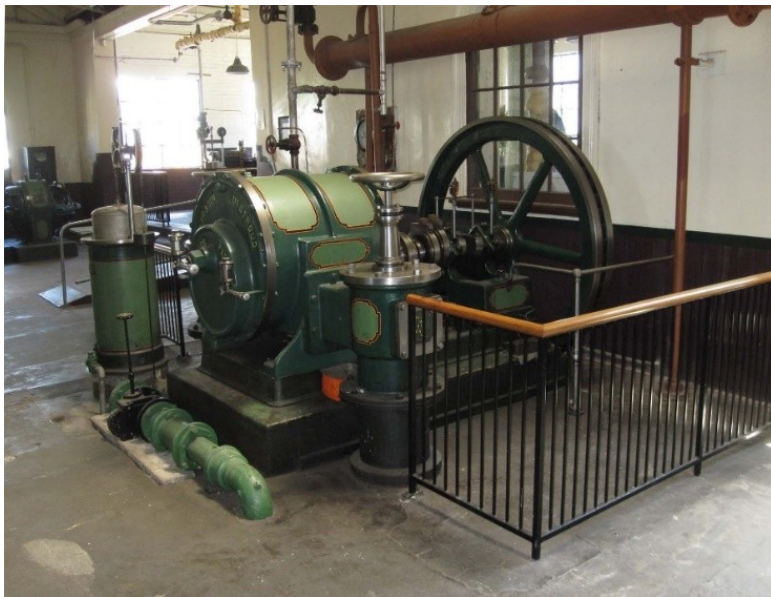
No 2 exhaustor, installed in 1939
