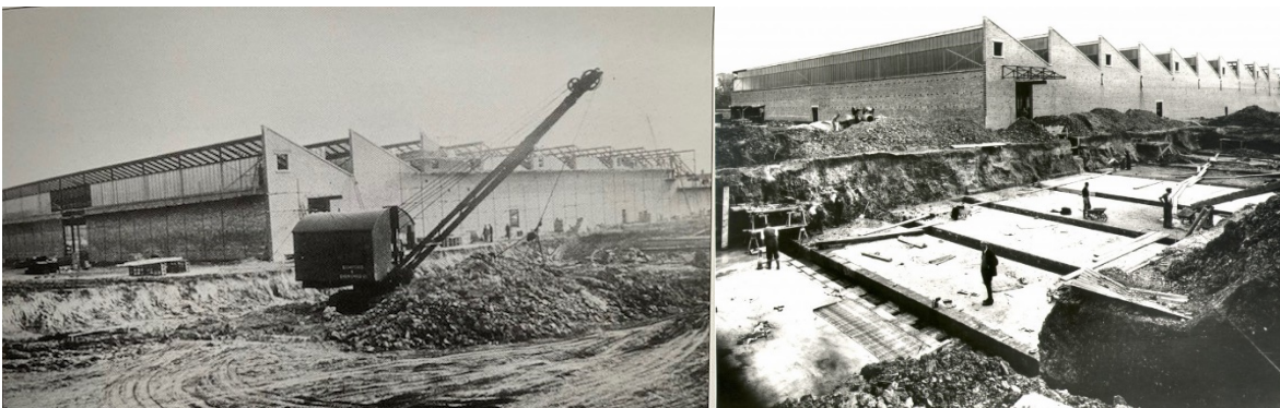
Photos showing construction of the main building and concrete footings being laid c1938
