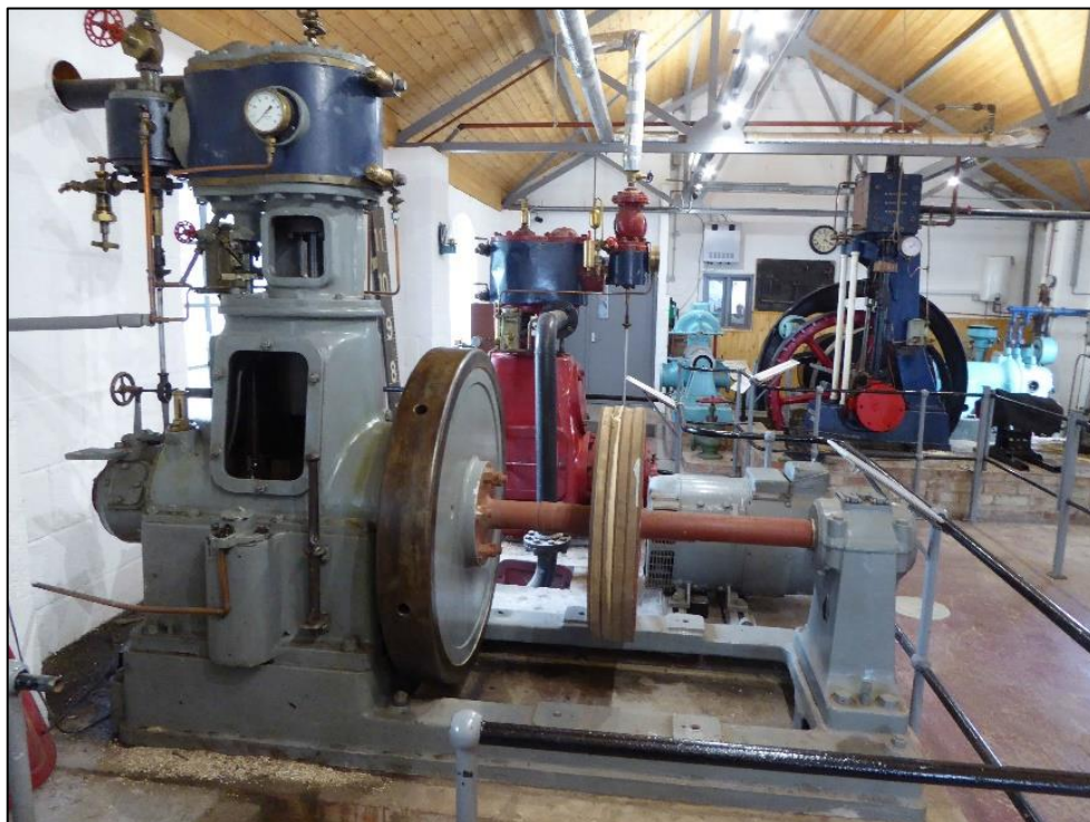
Fig 5. Electricity generation plant. Ex Stroud Hospital
