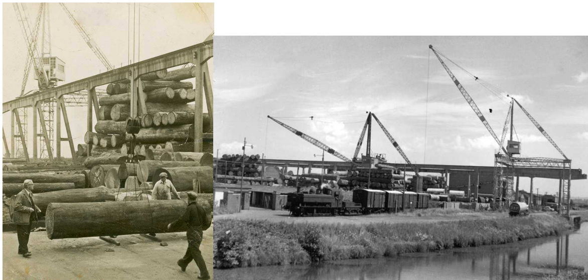
The gantry crane traversed Harbour Road, moving logs into the works
