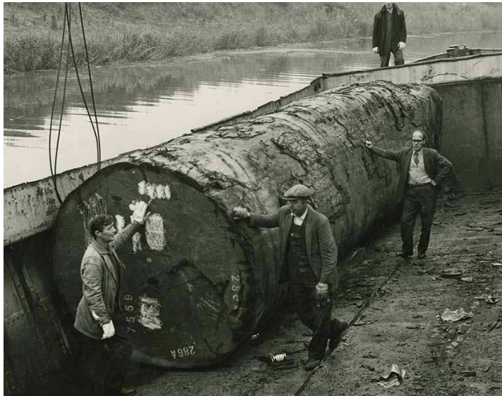
Timber delivery to the Pine End Works, reputedly the biggest log delivered by barge to Lydney
