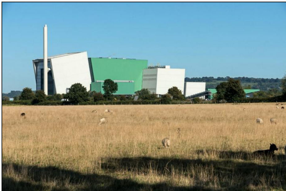
Javelin Park waste-to-energy plant (courtesy UBB)
