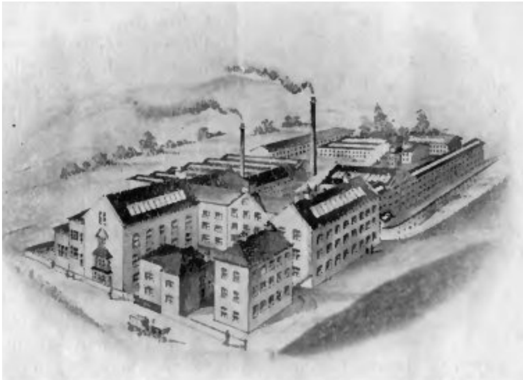
The extensive Dudbridge Mills site in 1910
