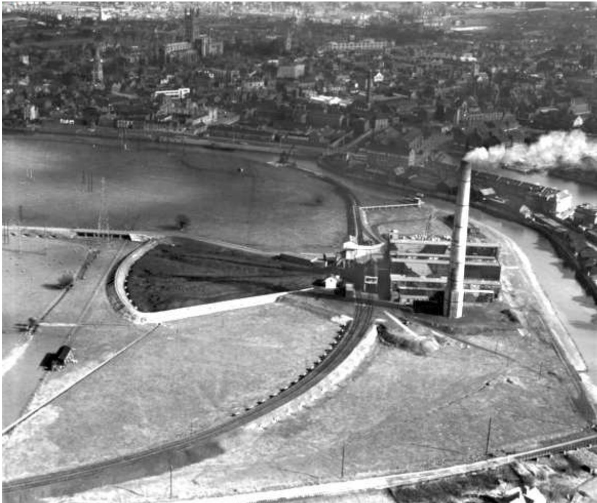
Two views of the power station in 1949, showing the rail link, coal stockyard, and proximity to the River Severn (courtesy Britain from Above series)
