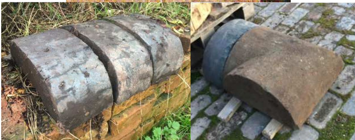
The Flat-topped blue capping bricks and a sandstone corner coping from the East wing of the station building, together with a matching half round capping brick. The upper photograph shows the stone corner coping in situ, with the dentil course clearly visible below.
