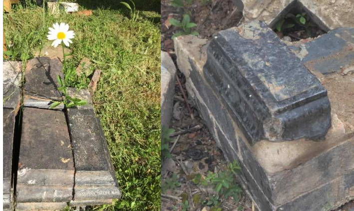
Some of the recovered blue string course bricks used at plinth level
