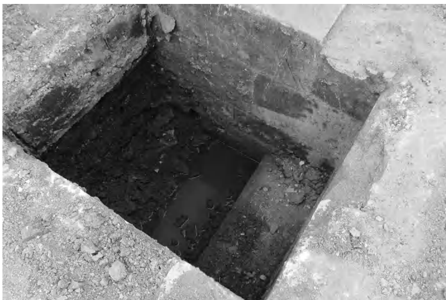
Figure 5. Excavation between two of the engine platforms showing the depth of the stone foundations and the small access tunnel (filled with mud) running beneath them.
