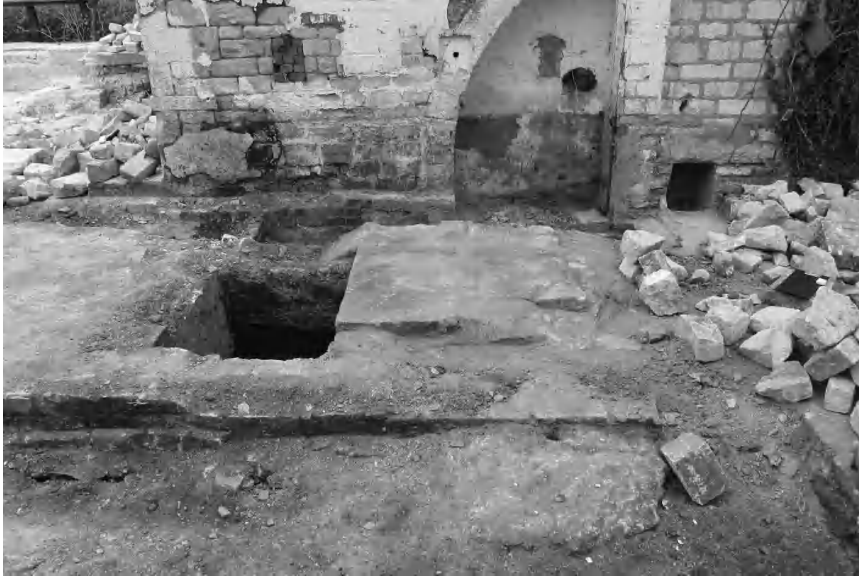
Figure 6. The surviving large stone platforms that carried the engine's main components.
