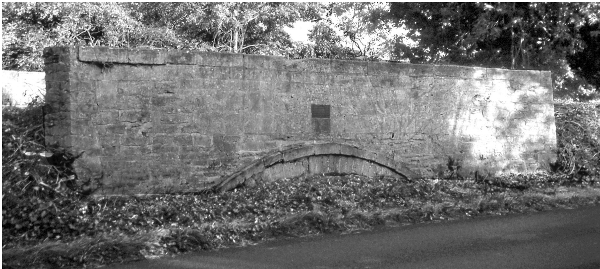
Fig. 1 The original A433 bridge over the Thames and Severn at Thames Head after the removal of undergrowth. The commemorative plaque above the arch reads :-
