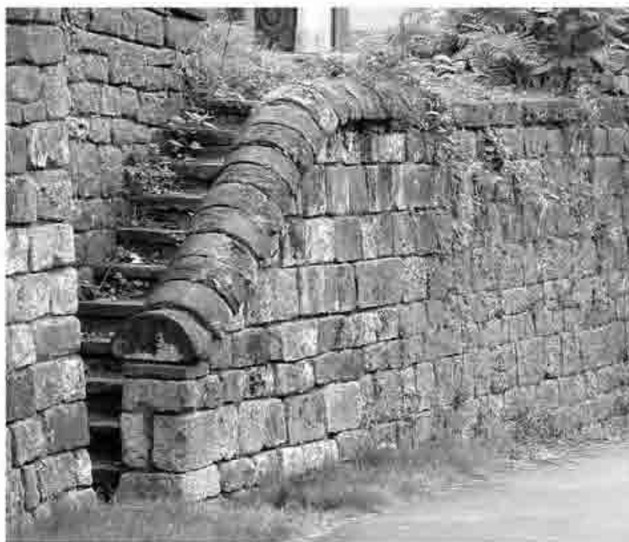
Figure 11. Half-round copper slag blocks being reused at Lower Redbrook
