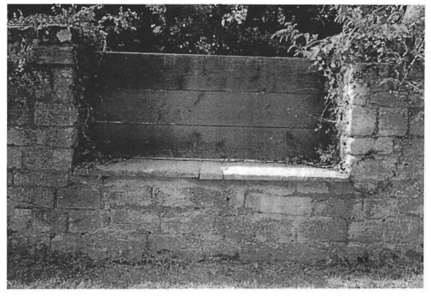
Figure 4 One of the Two Loading Chutes Fitted with Replacement Boards (Author)
