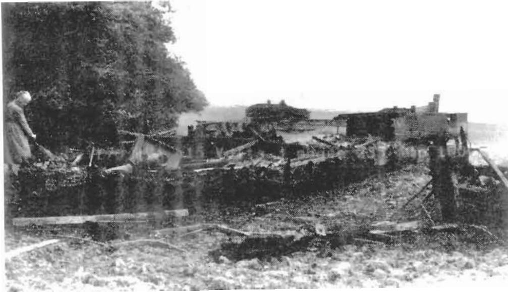
Above: The Severn Graveyard at Purton (22.6.86).
