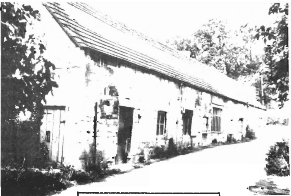
Brookhouse Mill 1982. (Savory's Pin Mill)
