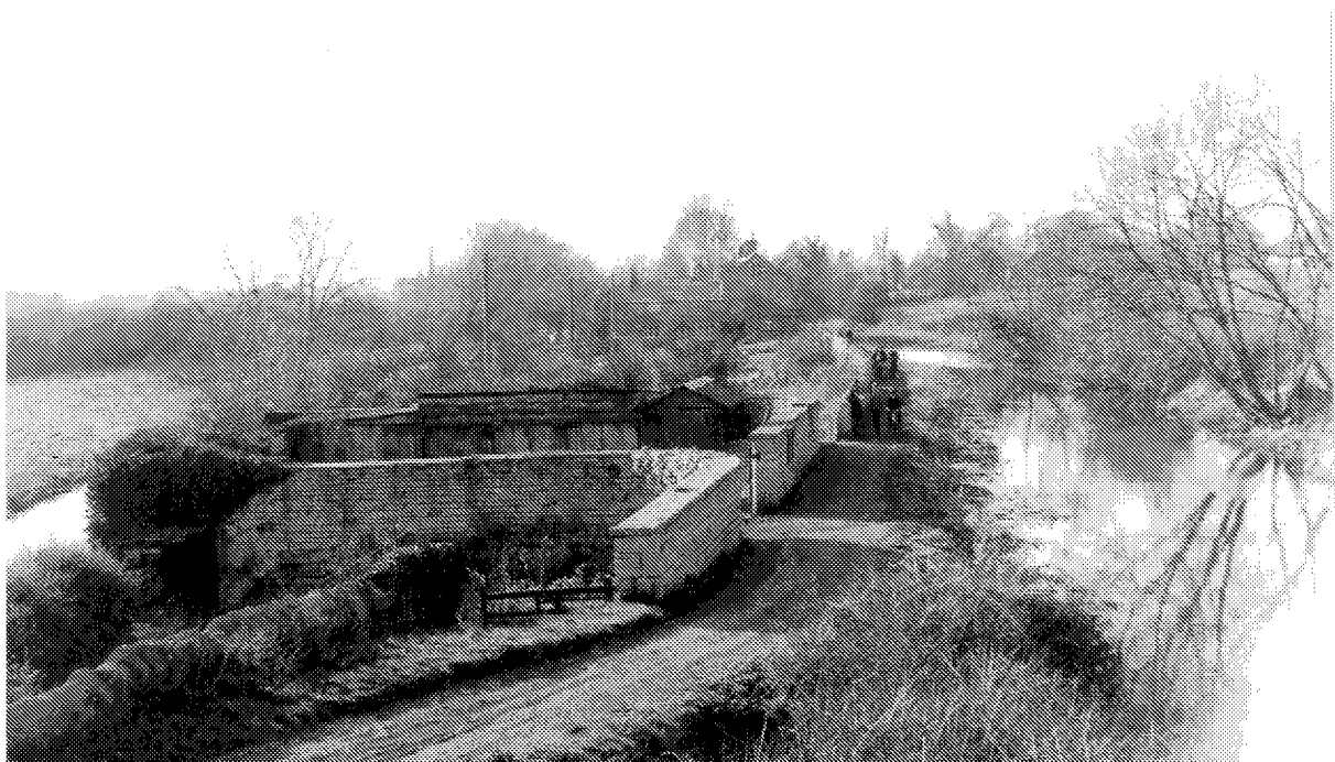
Figure 1 View of the Coal Pen Looking West Taken by Harry Townley in 1966
