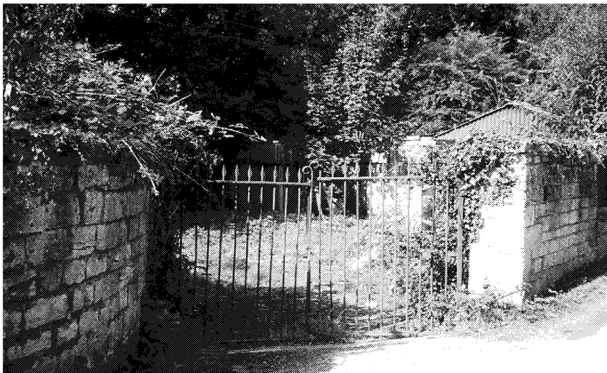
Figure 2 View of the Entrance to the Coal Pen in 2002, Looking South-west. (Author)
